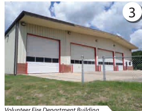
Volunteer Fire Department Building
