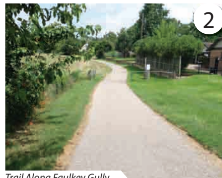
Trail Along Faulkey Gully
