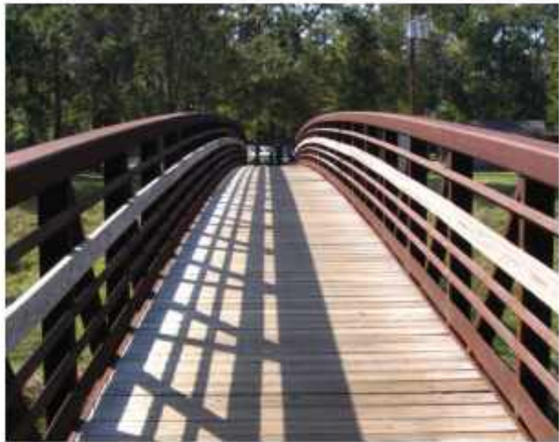
Pedestrian bridge at Faulkey Gully
