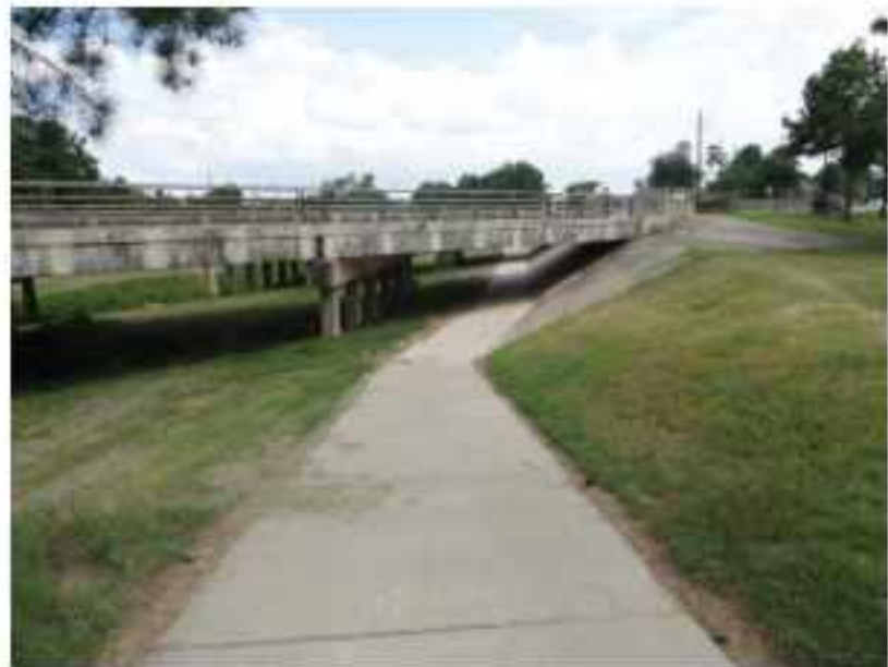
Existing Concrete Sidewalks
