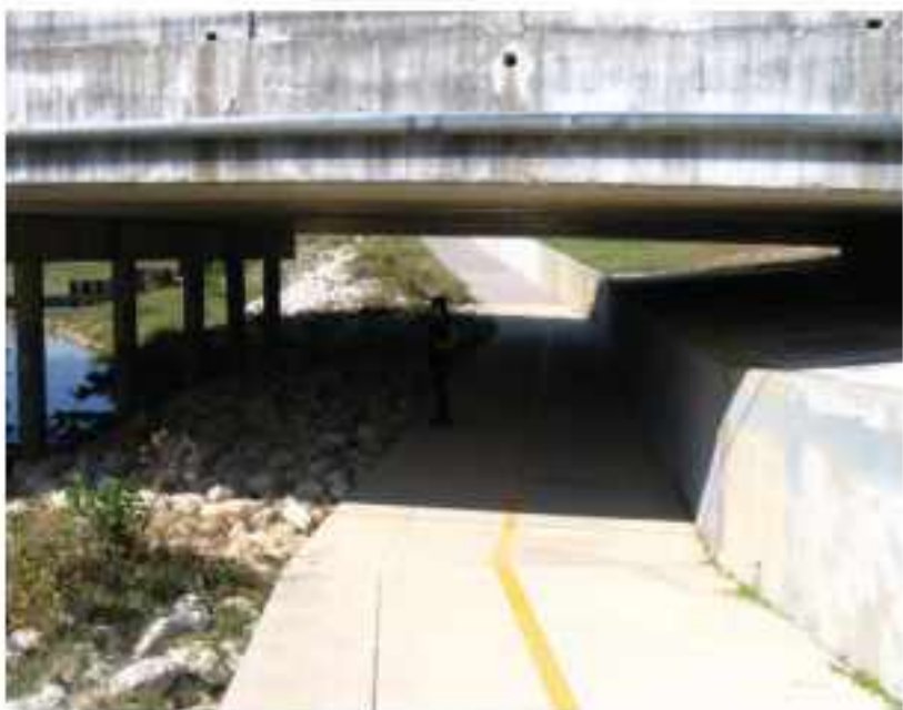
Undercrossing at Faulkey Gully and Louetta Road
